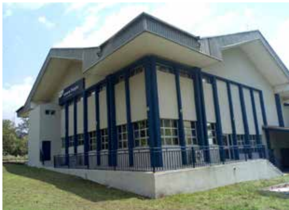
A renovated lecture theatre at the University of Ibadan as part of the Infrastructural Development Programme
